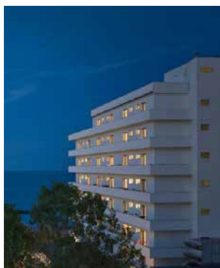
SERENA MAJESTIC HOTEL RESIDENCE Montesilvano, Italy bespoke fix and loose furniture + civil and MEP works for refurbishing of 215 guestrooms.
