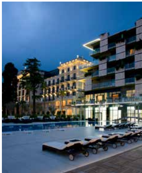
KEMPINSKI PALACE HOTEL Portorose, SI Refurbishment of the old + new building, 183 guestrooms and suites.
