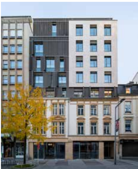
THE CENTRAL - APARTHOTEL Luxembourg, LU Supply of joinery and FF&E items for 28 luxury apartments.
