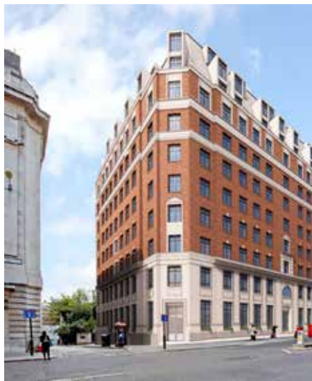
GREAT TOWER STREET London, UK Bespoke fix and loose furniture + civil and MEP works for refurbishing of 234 apartments.
