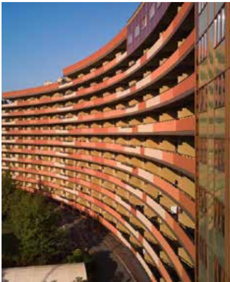
RIPAMONTI RESIDENCE Milano, IT Refurbishment of 850 apartments.
