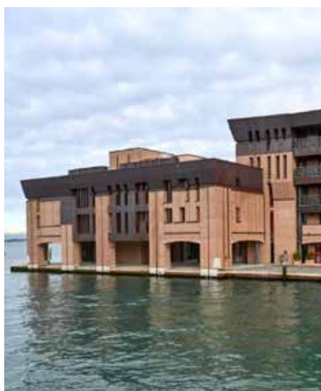
●RESIDENCE "SAN GIOBBE" Venice Dove Vivo Campus, IT Joinery and loose furniture for 230 guestrooms and public areas
