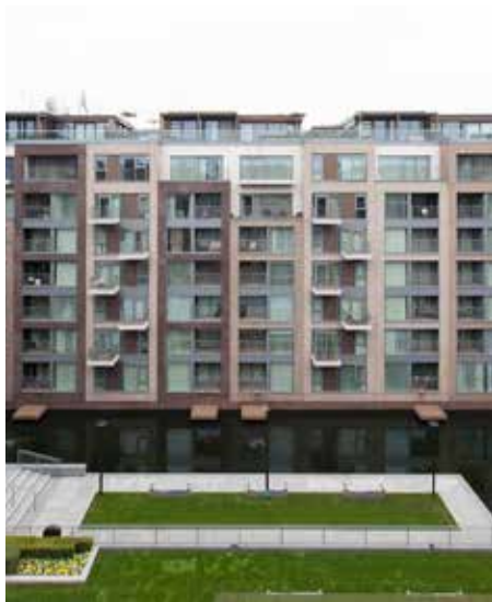
BURLINGTON GATE London, UK Wardrobes and dressing rooms for 42 apartments.
